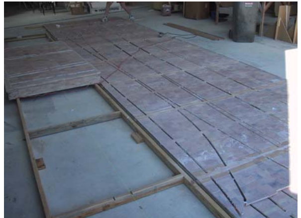
Pre-cut and pre-glassed panels of DuFlex—joined.
