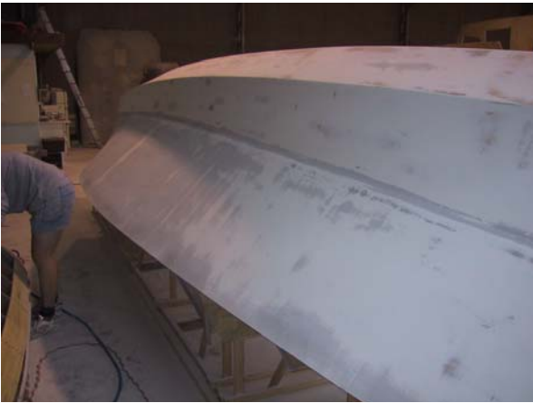
High Build undercoat sanded back.
