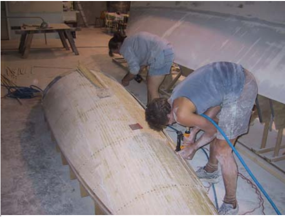
Cabin mold stripped up using durakore strips
