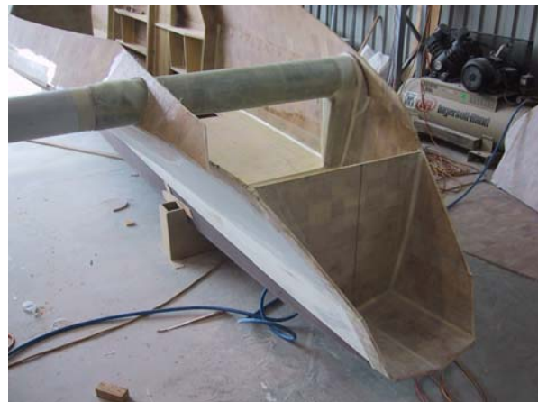
Aft beam socket.
