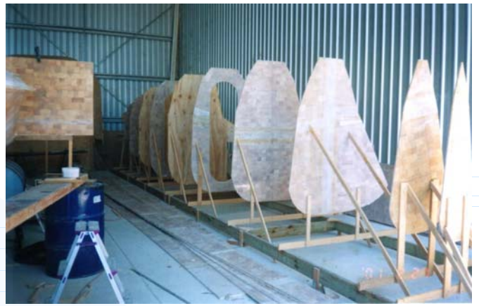
The bulkheads are stood upside down on a strongback. A couple of temporary frames are added.
